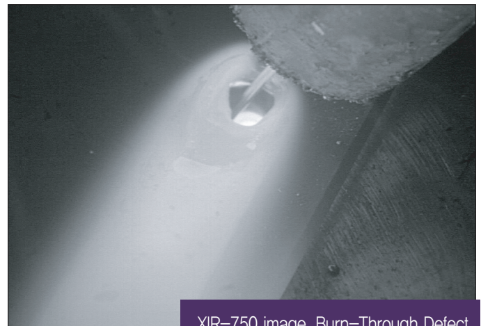
XIR-750 image, Burn-Through Defect
