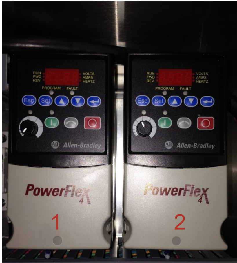
Figure 12 Variable Frequency Drives (VFD's): #1 for main conveyor motor and #2 for seamer motor
