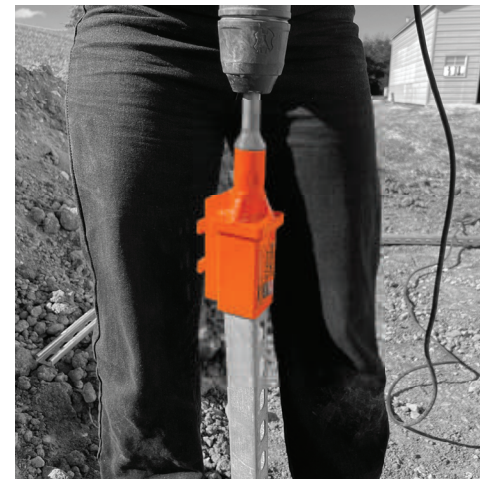
End receiver for driving from the top.
