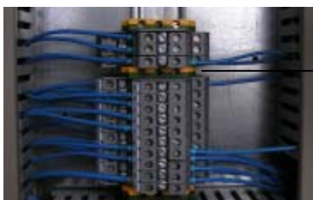
binding postes 24 V before EMERGENCY- Stop
