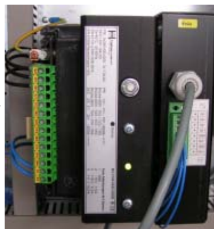
binding postes 24 V before EMERGENCY- Stop
