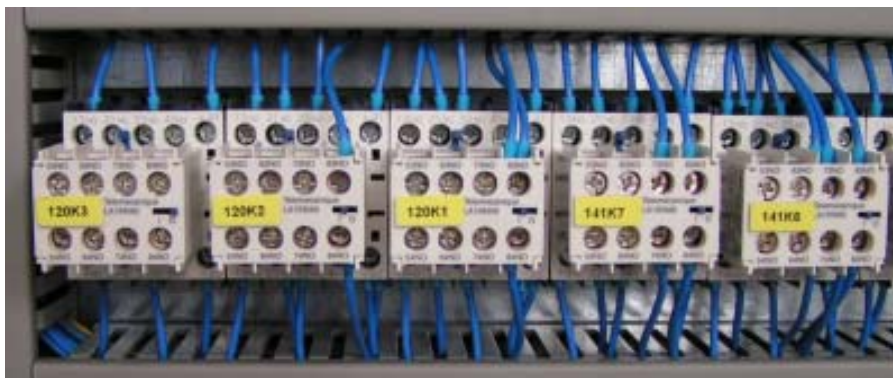
contactor relay
