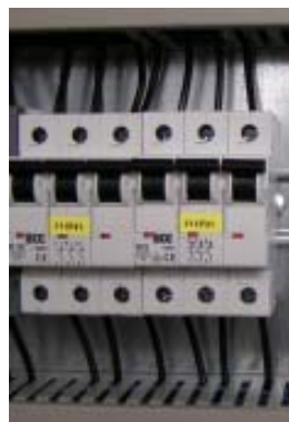
protected switch for drive
